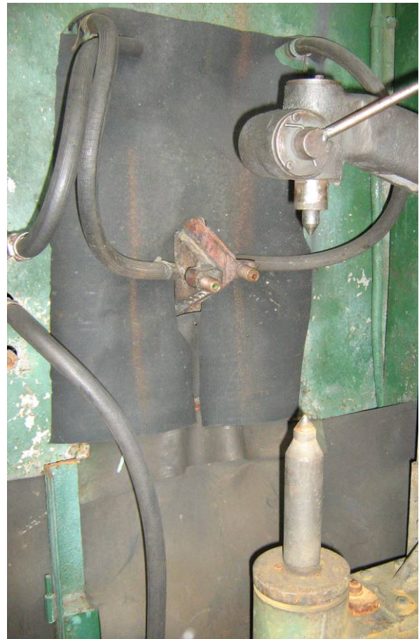
Fig.3. Workplace no.2 of heating installation IMCA-2-110E.
